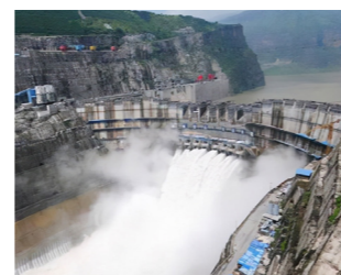
Hydroelectric Power Plant
