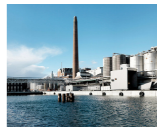
Local Heat Supply Plant
